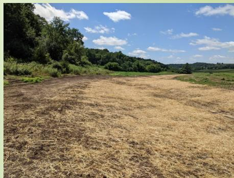
*Pictured to the left is a 2,500 linear foot grassed waterway serving as a drainage area for 258 acres in Section 25 of Spring Grove Township.*
