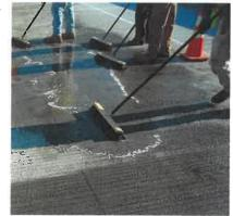
T-78 Polymer Crack Sealer seals cracks effectively and can be open to traffic in as little as an one hour.
